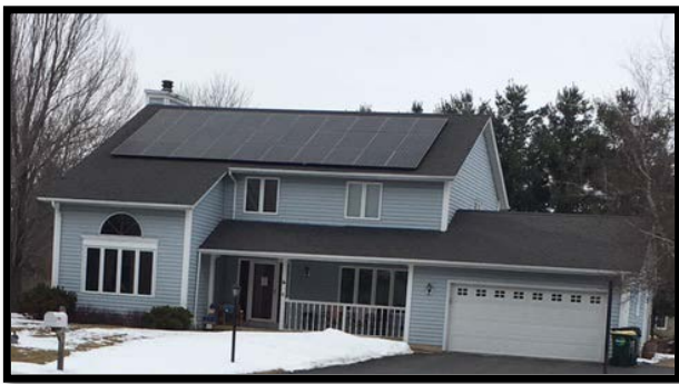
Note: a roof mounted solar energy system located on the front of a home or accessory building and installed in a uniform pattern requires a variance.
